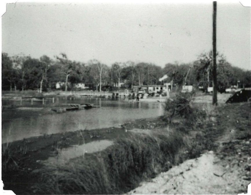
Red Bluff Road, old and new bridges over Taylor's Bayou, 1971
